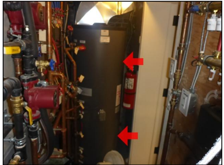
Indirect fired water heater
