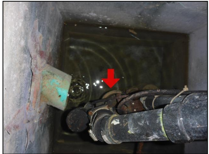
Sump pump (submersible type)
