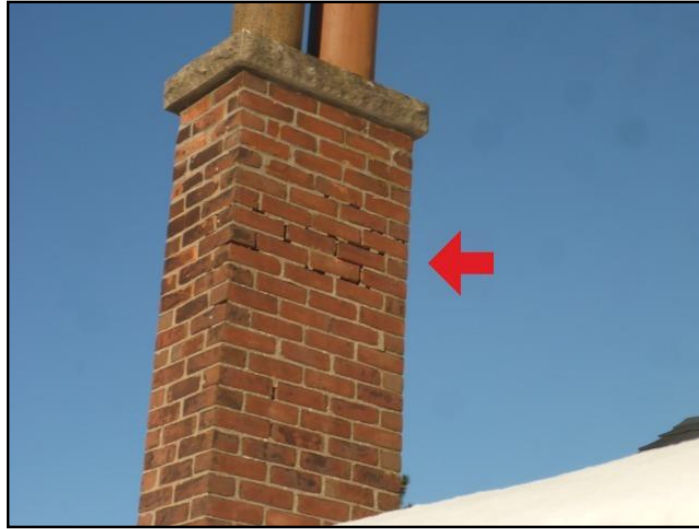
Loose, missing or deteriorated mortar
