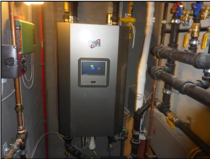
Integrated (combination) system- boiler
