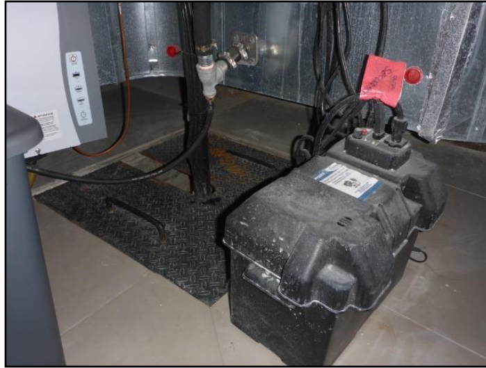
Batter powered backup pump noted
