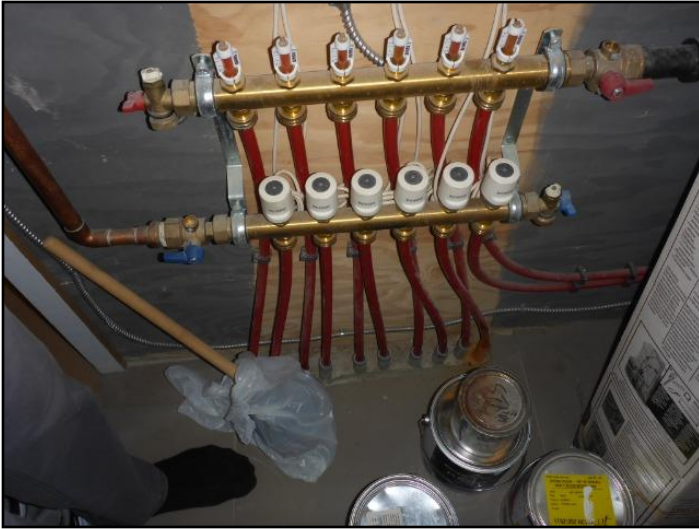
Radiant floor heat (typ.)
