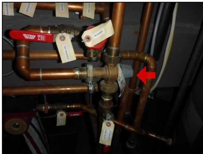
Tempering valve may need adjustment
